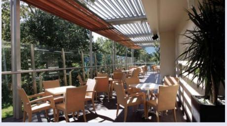
Acoustic issues were overcome by incorporating 1.8-metre high shatterproof glass panels which minimise noise levels to the public park without losing the view.
